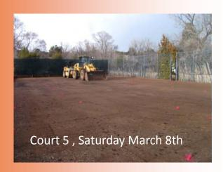
The old surface on Court 5 has been removed. By the time you read this Court 5 will be paved with new asphalt. The asphalt needs to cure for about 2 to 4 weeks before the tennis court paint can be applied. Painting the court takes a few days. That means new court could open as soon as early April. Then work will begin on the next hard court.
